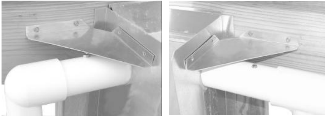
Figure 14. End Panel Support Installation
